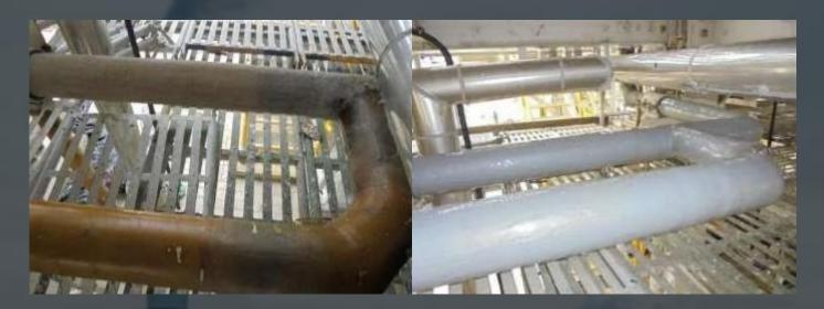
**DENSIQ Liquid Insulation Composite coatings are** based on a combination of innovative fillers bound in protection for metallic surfaces and reduce the a 100% solids epoxy resin.
