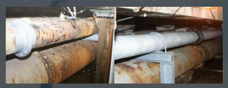
DENSIQ composite pipe repair products can be used to seal leaking pipework ranging from 1/2" (1.2cm) to 48" (121cm).
